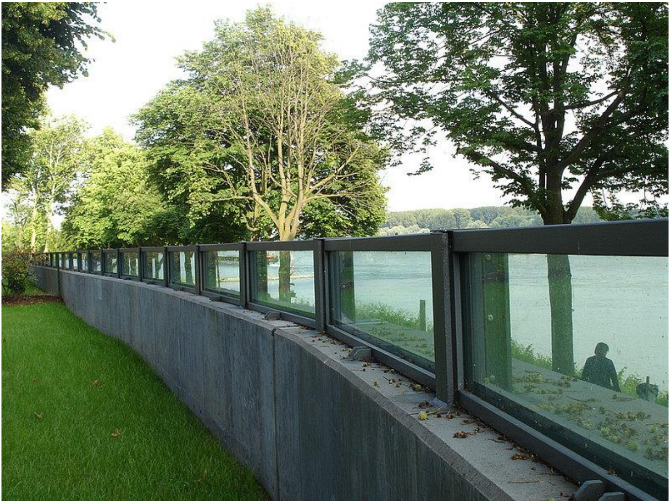
Cologne has built flood walls to protect the city for when the Rhine floods
